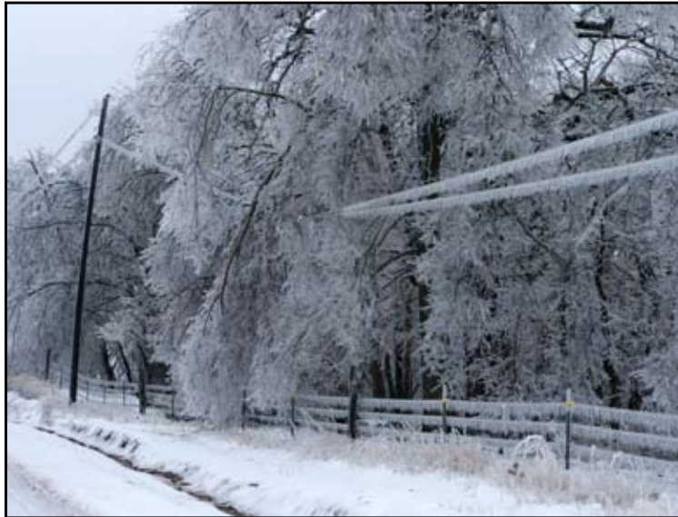
Layers of ice coated tree limbs and Brown-Atchison's power lines in the December storm, causing a complete system outage for the co-op.
