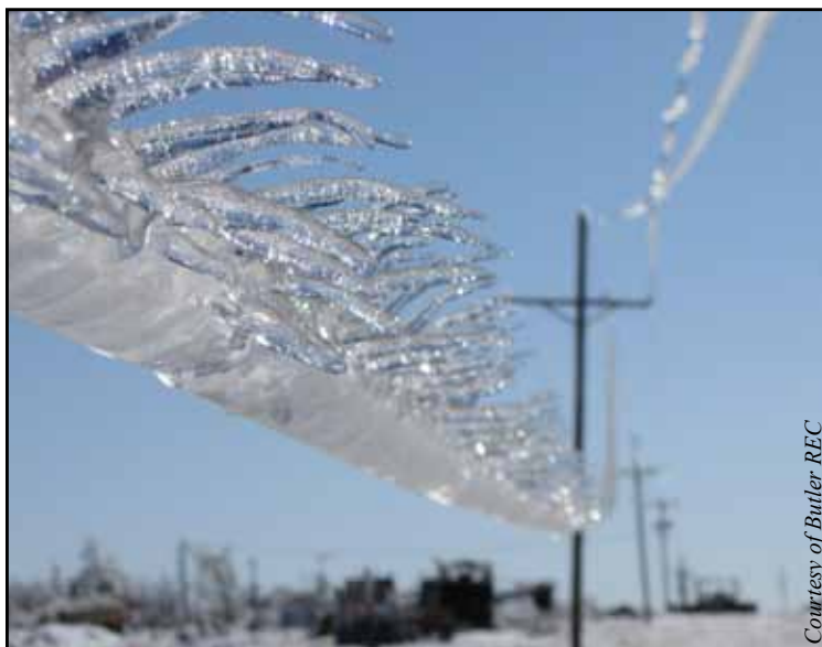
Ice coated power lines on Butler's system in a winter-like storm on March 27, 2009.
