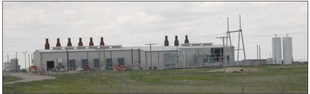
Midwest Energy's Goodman Energy Center began commercial operation last month northwest of Hays. The 75 megawatt gas-fired facility will be used to meet peaking needs.
