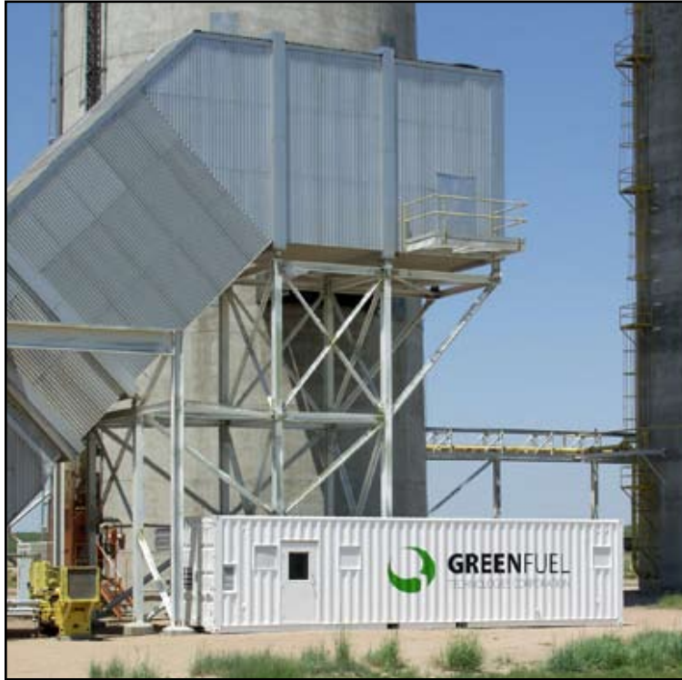
The developer for Sunflower's algae farm subsystem, GreenFuel Technologies, delivered a mobile laboratory to ensure that flue gas from the Holcomb plant can be used to grow microalgae in an enclosed environment.
